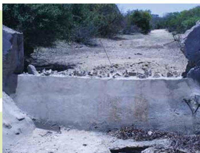
A sand storage dam built by stages of reduced height in Zimbabwe is a perfect example of a design innovation which has the potential to increase the capacity of the sand reservoir to supply water. Source: De Trinchiera, 2015
