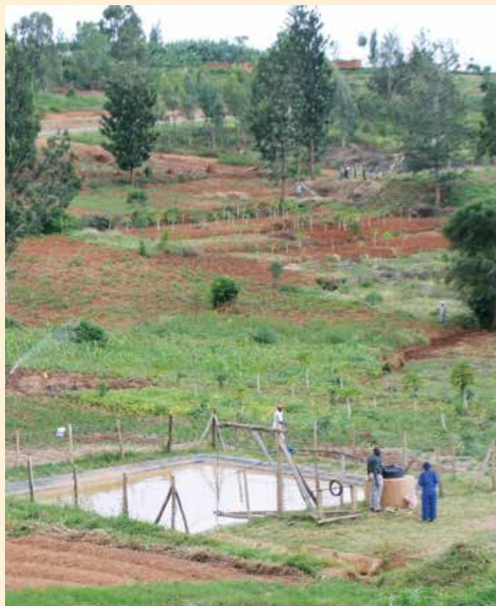
*A RWHI system based on a farm pond is complemented by other micro-catchment and in-situ RWH management technologies. Source: Oduor, 2015*
