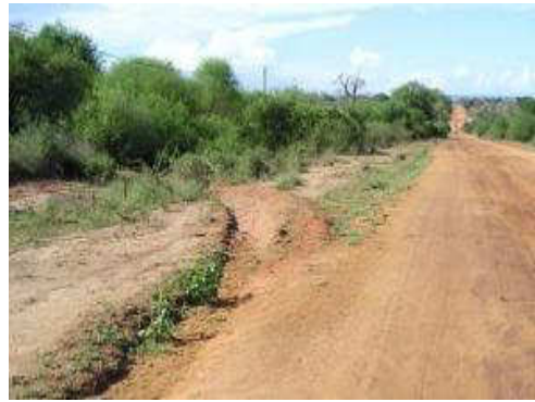
Figure 5. Roadside diversion ditches can be used to collect runoff water which can collect in roadside ponds. Sources, E. Nissen-Petersen, Kenya.
