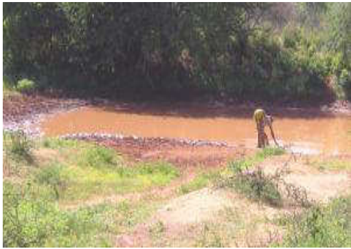
Figure 5. Roadside diversion ditches can be used to collect runoff water which can collect in roadside ponds. Sources, E. Nissen-Petersen, Kenya.
