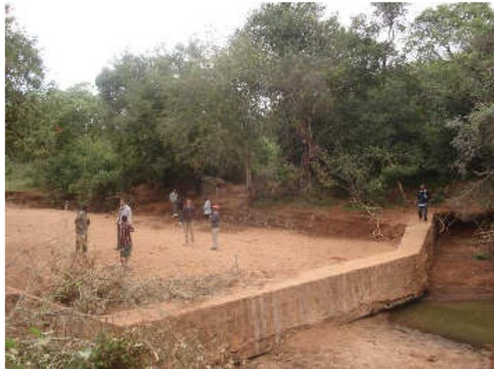
Fig 2: Sand dams constructed along intermittent stream in Yabello, Borana Zone of Oromia Regional State (Photo: Amare, 2011)
