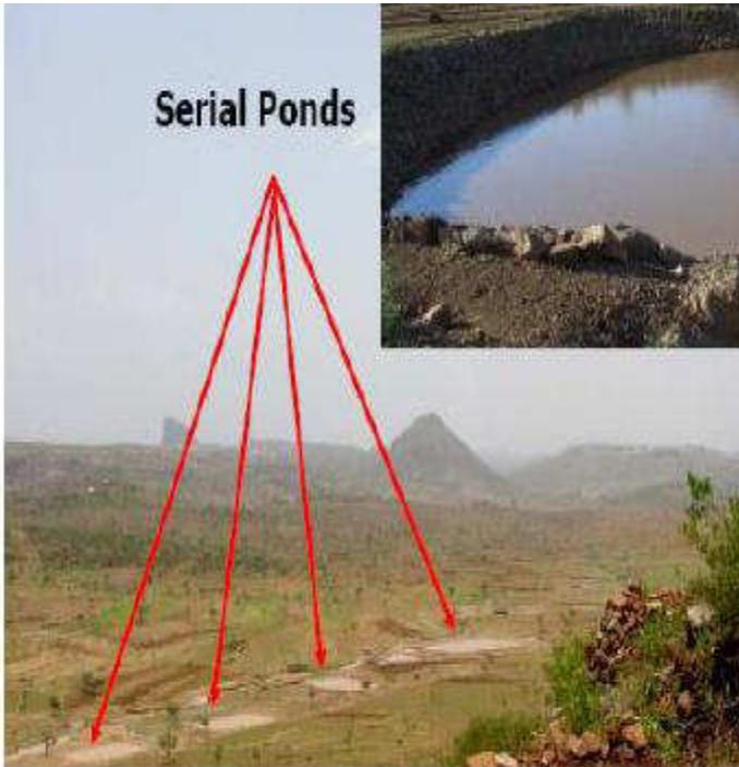
**Fig 1a serial ponds constructed in a gully**
