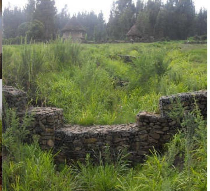
**Fig.1b. Sediment harvesting in a gully**
