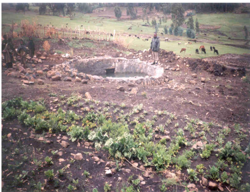
Figure 1: A stepped tank is used to provide water during the dry season to an irrigated crop area in Ethiopia
