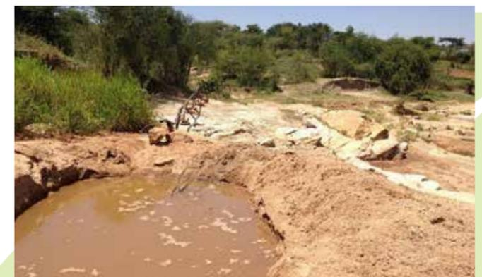
Sand storage dam connected to a small-scale irrigation system in Machakos (Kenya). Source: AFRHINET project
